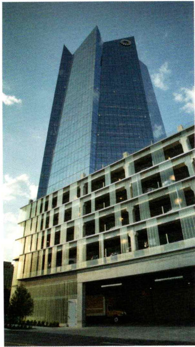
Frost Tower Parking Garage San Antonio, TX
