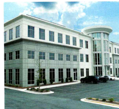
New Hope Medical Office Building Duluth, GA
