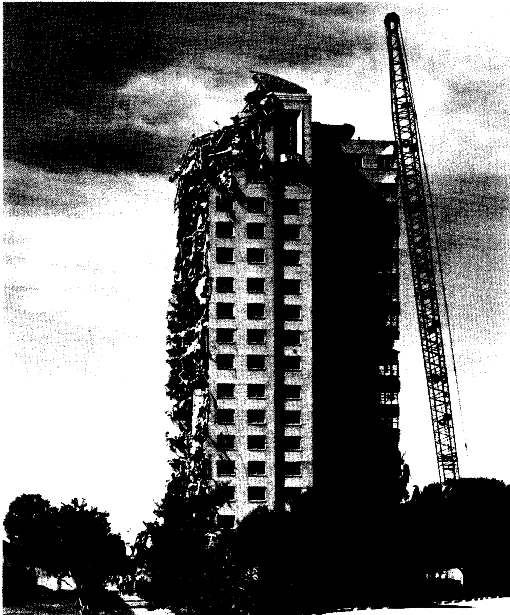
Above Shamrock Hotel Demolition, Houston (1987).
