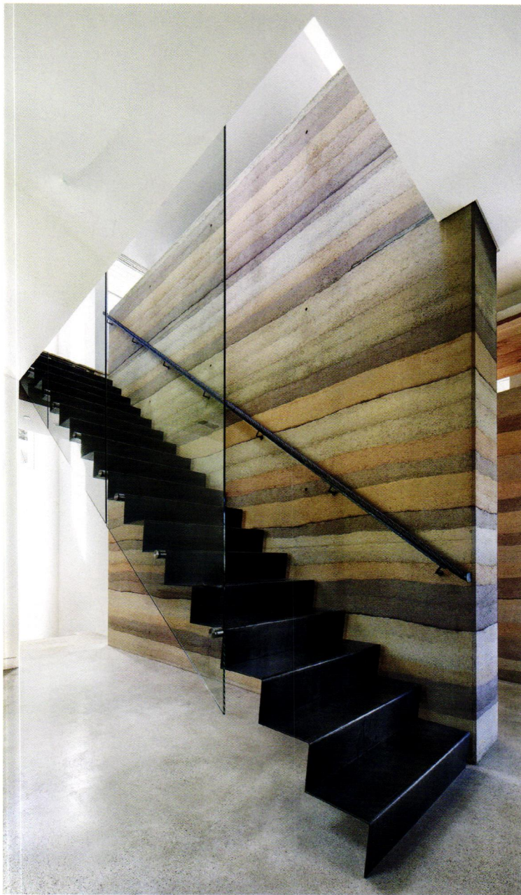
The Sundown Residence, by Mark Oberholzer, AIA, with Glass and Dangel, utilizes graphic rammed earth walls throughout. “Mockups had to be made to determine color, texture, proportions, and dimensions. The design process was iterative and almost more like a design-build process,” says Uli Dangel, AIA.
