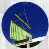
prefabricated exterior wall panels
