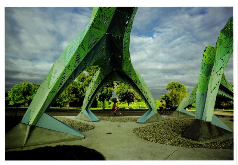
Above Pre-cast concrete buttresses provide a durable support and resolve in an architectonic detail how the work meets the ground. Right The interlaced structural elements are reflected in plan as hardscape, divided into paving, greenspace, and paths around the work.
