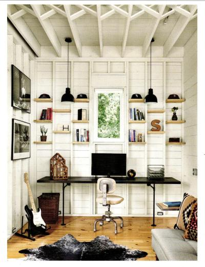
Left With the cladding, insulation, and weather seal all outside the structure, the architects were able to leave the framing exposed on the interior. Below The lack of large overhangs allowed the house to be completely wrapped with a water, air, and vapor barrier, making for a very tightly sealed envelope. The corrugated metal siding and standing seam roof are typical of East Austin.
