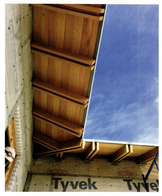
Above FP&C leaves its mark with refined details, such as the paired fir outriggers, which will be set apart from the heavy-dash plaster with clean reveals.
