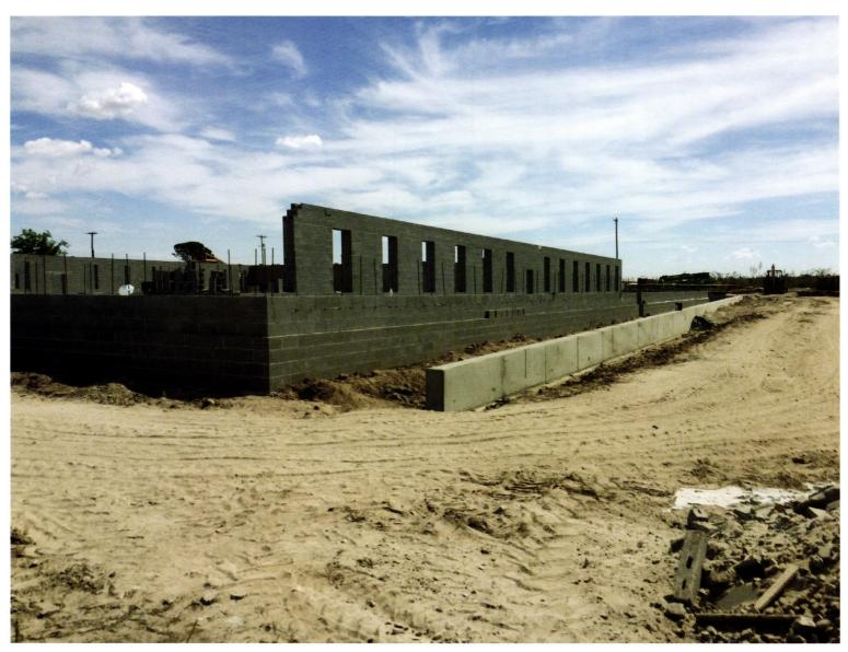
A substantial cast concrete retaining wall allows the building to sit on a flat plane set into the sloping 3-acre site. Extensive subsurface drainage systems handle occasional torrential rains. purpose. "Somewhere, a portion of contemporary art has to exist as an example of what the art and its context were meant to be," Judd later wrote. Irwin and Judd discussed their work, then parted ways. This chance encounter would be their first and only meeting in Marfa, Texas.
