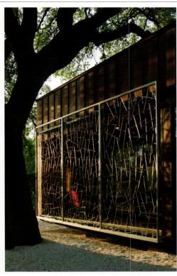
**Left** To get the house as close to the tree as possible, the architects cantilevered the structure 9 ft from its last pier. A stainless steel screen offers a bit of geometric relief from the otherwise orthogonal building.
