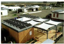
6kW PV array powers the house, which is also equipped with a rainwater catchment system and an aquaculture and permaculture garden for growing food.
