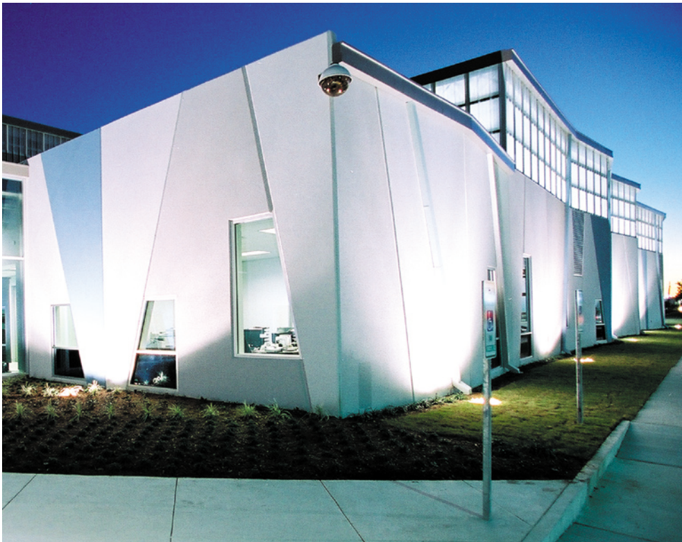
The MNP Corporate Headquarters in Houston, designed by Powers Brown Architecture, utilized tilt-wall construction to achieve a skin that suggests a billowing surface.
