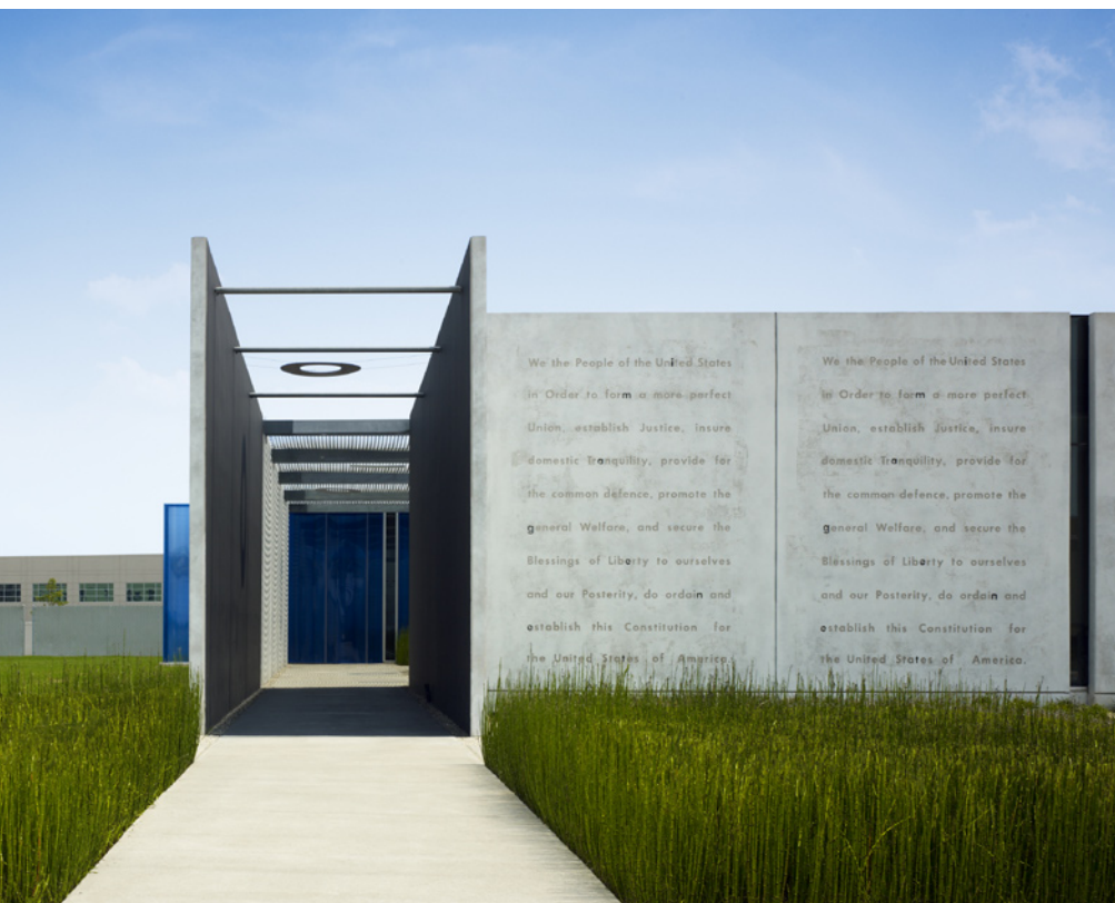
(above) Tilt wall construction was used in the design of the ImageNet Houston building by Elliott + Associates Architects. The project emphasized economy and expandability. (below) The Pickle Elementary School/Virginia Brown Community Center, designed by TeamHaas Architects now Nelsen Partners, incorporated concrete tilt-wall panels which form the spine of the building. Window and door openings were created by the edges of the panels, simplifying formwork and fabrication time.
