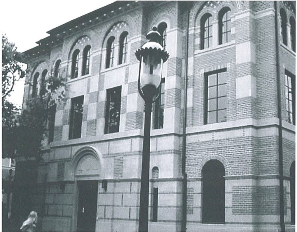
Rice Humanities Building, Rice University; photo courtesy Texas Masonry Council
