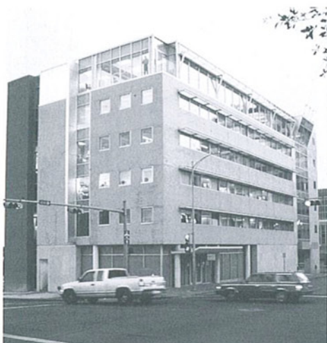
Renovation & Addition: 1011 San Jacinto Office Building
