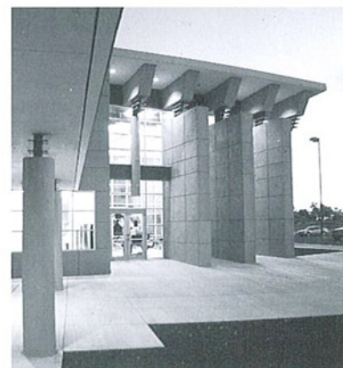
El Paso County Juvenile Courts Facility
