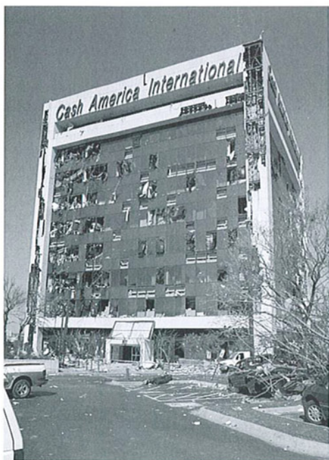
(above) Detail of the Cash America International building. (below) The building was heavily damaged by the 2000 tornado. (right) Rendering by Carter & Burgess of the restored building. Photos and rendering courtesy Carter & Burgess.
