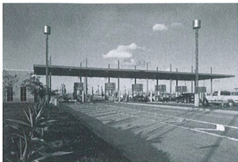
Los Tomates Toll Station & Administration
