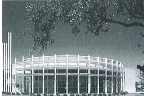
Frost Bank/De Zavala Branch
