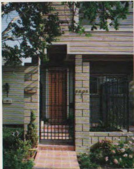
raised landing of the stair, required to satisfy the building code requirement of no continuous vertical run more than 12½ feet, allowed the creation of a recess above the front door in the soffit of the second-floor overhang—possibly to be read as an allusion to a ceremonial entry portal.
