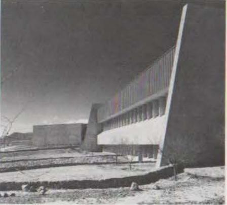
*Vertical fins and deep recesses reduce heat load.*
