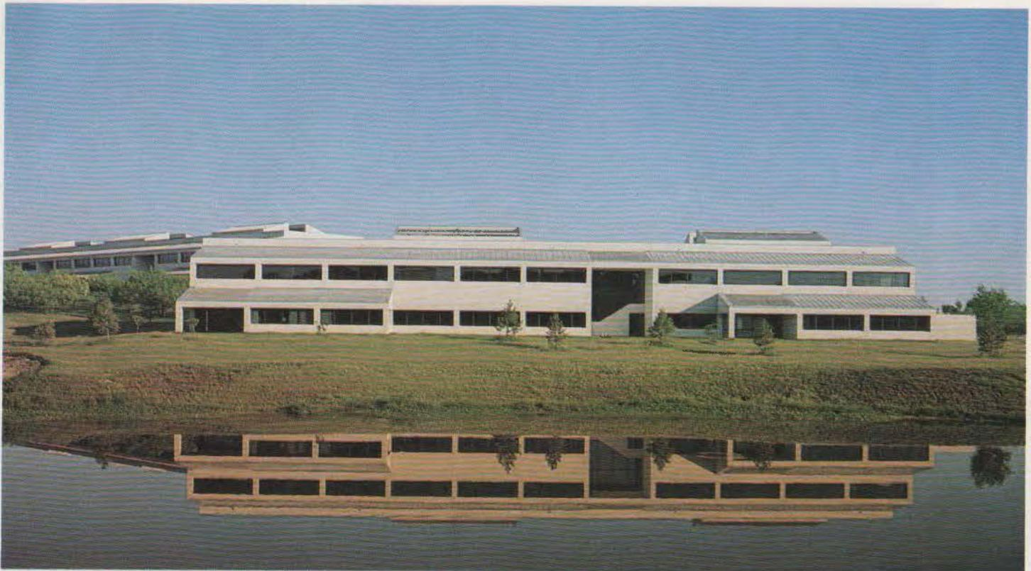
perimeter bays hung like saddlebags from each side of the box. Their sloping shed roofs are of standing-seam metal, with cedar trellises over glass areas where the glazing extends from floor to ceiling. The sloping roof motif is repeated on the flat roof of the box by "sheds" covering the conventional mechanical equipment, to shade as well as hide it when a high-rise goes up nearby. Recessed windows are of tinted glass, and the exterior finish is stucco.
