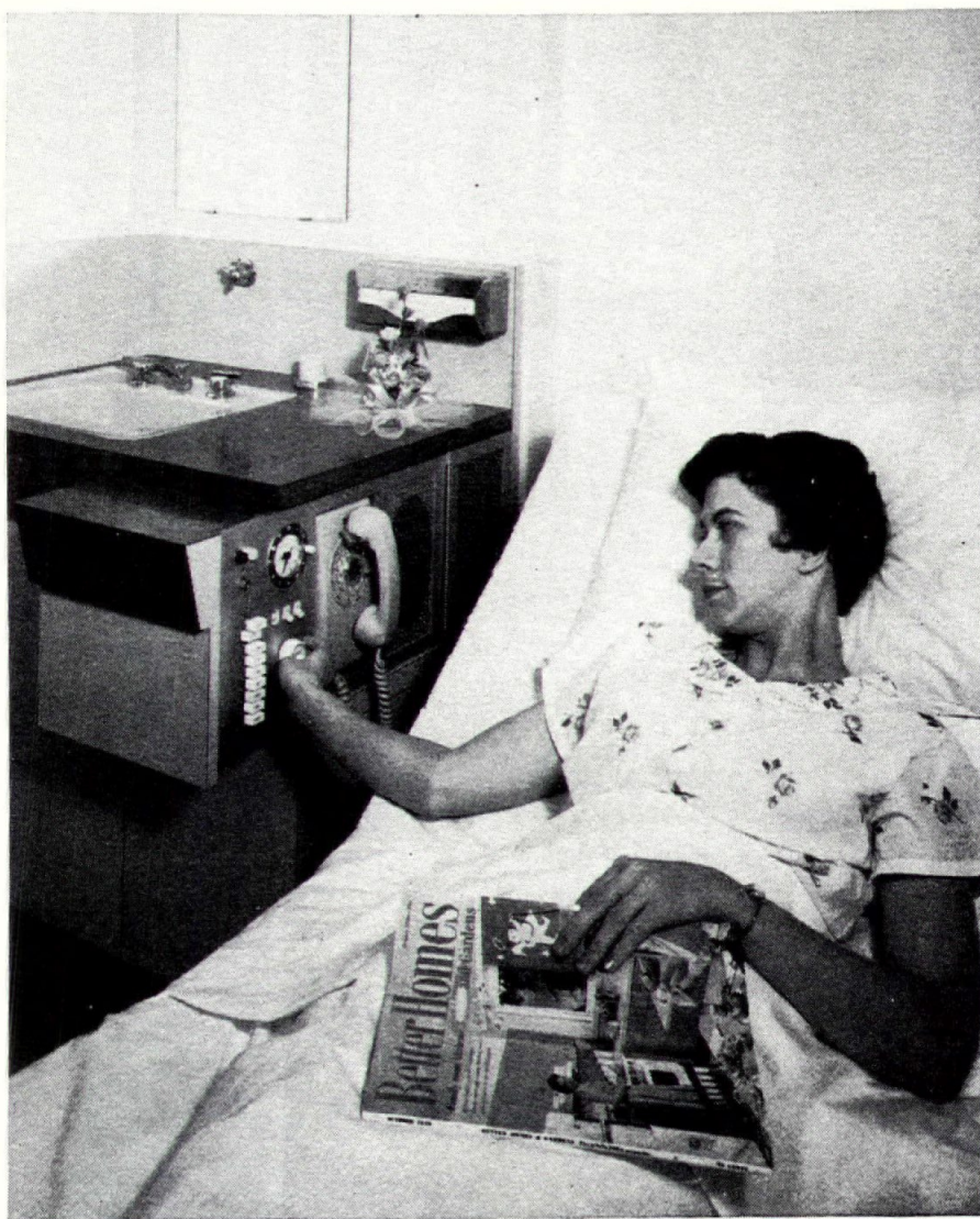
Built-in bedside unit is a combination wash stand and control panel. Within easy reaching distance, the patient can control television, radio and music, set the clock, call the nurses' station, use the telephone, flip an overhead light.
