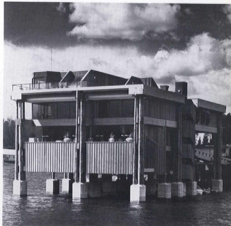
The lake side view of the Hagedone Offices . . . the cluster of cedar log piling columns support the glulam beams and is characteristic of all the interior supporting columns.
