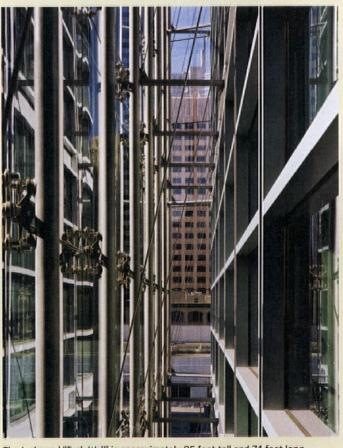
The L-shaped "Tech Wall" is approximately 95 feet tall and 74 feet long. Horizontal mullionless, point-supported glass provides the outer facade. These structural glazing panels are attached to vertical tension trusses, creating a four-foot cavity.
