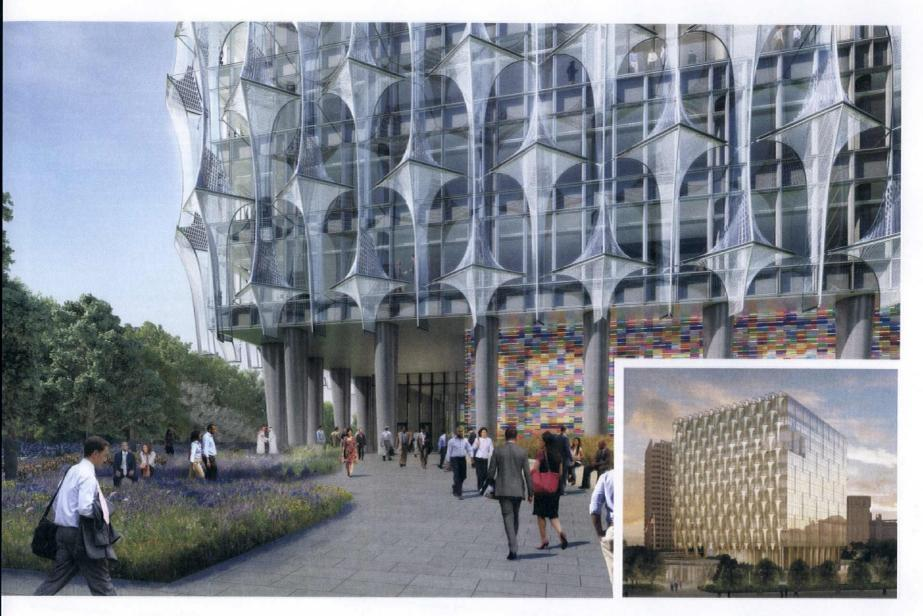
lattice, made of ethylene tetrafluoroethylene (ETFE) film, projects from the building's curtain wall to reduce solar gain, cut glare, and admit an even, diffuse daylight, while still allowing occupants generous views of London. Photovoltaic cells on the skyward surfaces of the ETFE elements will harvest solar energy, and the entire assembly will interrupt downdrafts, making for more comfortable outdoor spaces below. Not least, the outer envelope is intended to deter bird strikes.
