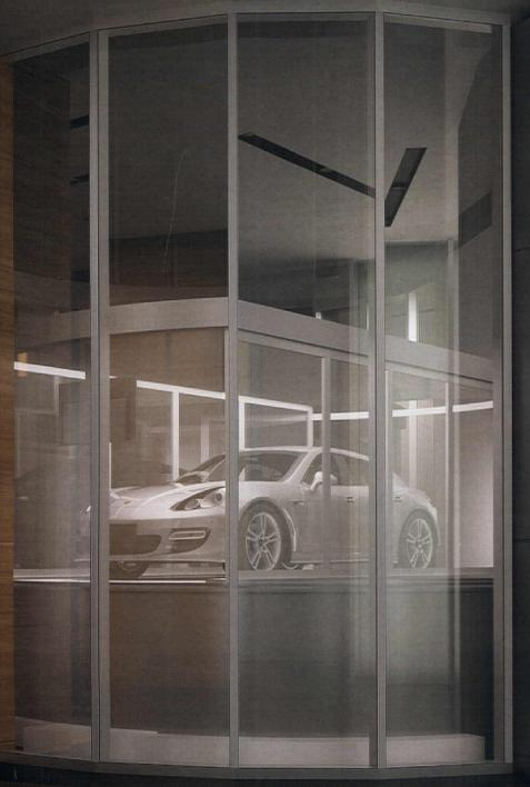
2 HOUR FIRE RESISTIVE **GLASS ELEVATOR ENCLOSURE** WITH SUPERLITE II-XL 120 IN GPX CURTAIN WALL FRAMING
