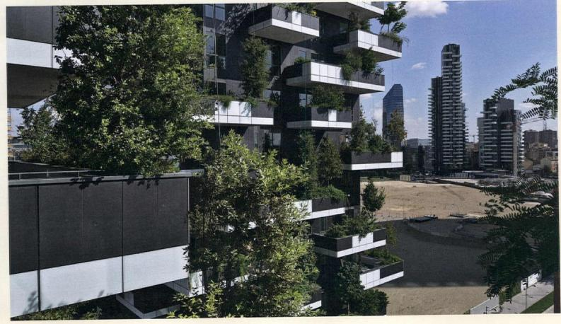
containers in which the plants grow—which measure over 5,500 linear feet in total—is the responsibility of the condominium. Larger plantings are secured with thin vertical cables.
