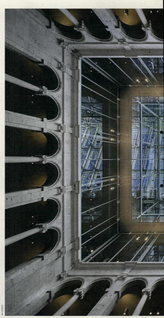
The facility's center, within the restored travertine Calderwood Courtyard, was extended upward with glass arcades on the top three floors and a new glass roof.
