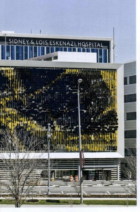
TWO-FACED Each of May-September's 7,000 folded-aluminum panels is finished in two colors of Durethane; the east-facing flaps boast a golden glow while their west-facing brethren are indigo.
