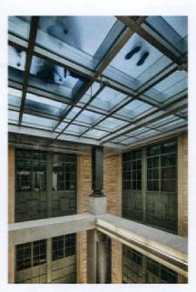
SHINING THROUGH Flad Architects used TGP's translucent Fireframes ClearFloor System to allow daylight to penetrate from the fifth floor to the ground floor of Northwestern University's new Engineering Life Sciences building.
