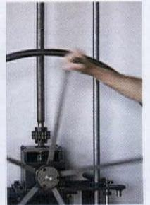
**OPENING ACT** At 242 State Street in San Francisco, Tom Kundig custom designed the exposed door-opening system that operates a 16-by-10-foot guillotine storefront (left). The hardware components (above) are constructed of waxed raw steel.
