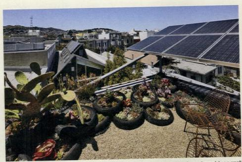
The insulated roof, protected by a drainage mat, weed barrier, and gravel, has a small seating area where succulents grow in planters made of old motorcycle tires.
