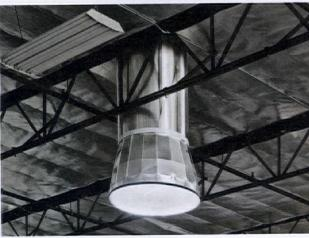
TRICKLE DOWN SkyVault Series Collector (top) and SkyVault Series Amplifier (above) catch and reflect light down into interior spaces.
