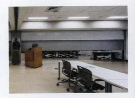
**SUMMIT® VERTICAL LIFT PARTITIONS SNAP 62** With the touch of a button, the panels in this innovative retractable wall system cascade down through a narrow slot in the ceiling, quietly sliding into place, and rise to store above the ceiling when not needed. Optional full-width writing surfaces are available.
