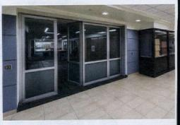
ACOUSTIC GLASS WALL PARTITIONS SNAP 6 Hufcor's acoustic glass wall achieves up to 44 STC and can be supplied with inset pass doors to allow easy egress and expandable closures to seal them tightly into place.
