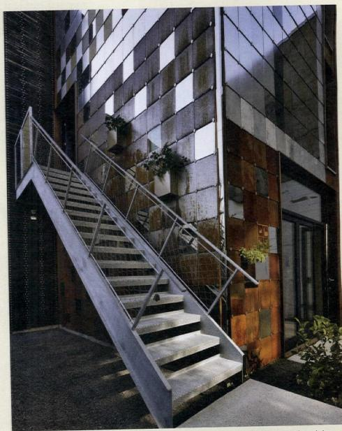
For the custom rainscreen, shingles made from salvaged metal and mirrored glass are held in place with clips and caulk strips.
