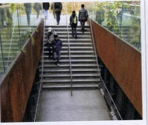
**KEEP WALKIN**<sup>2</sup> In appropriate design locations, slip-resistant metal can enhance the safety of walkways and stair treads.
