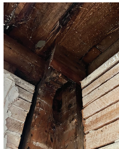
The main 8- by 8-inch corner post had been roughly shaped by hand.
