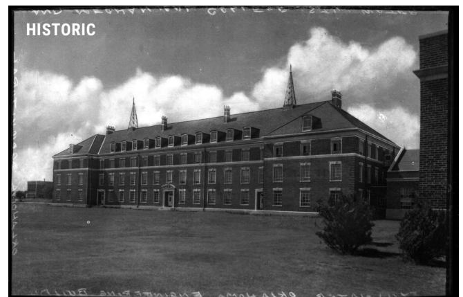
BEFORE/HISTORIC PHOTOS: Rand Elliott Architects
