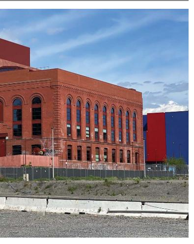
▲ The **NEW BOILER HOUSE** is clad in washed red concrete, an economical material that is sympathetic to the brick of the turbine hall while remaining true to its modern expression.
