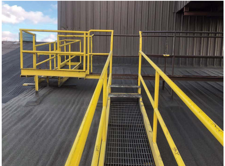
AN ACCESS WALKWAY AND ITS POSTS AND PENETRATIONS WERE SEALED WITH THE RE-COVER SYSTEM.
