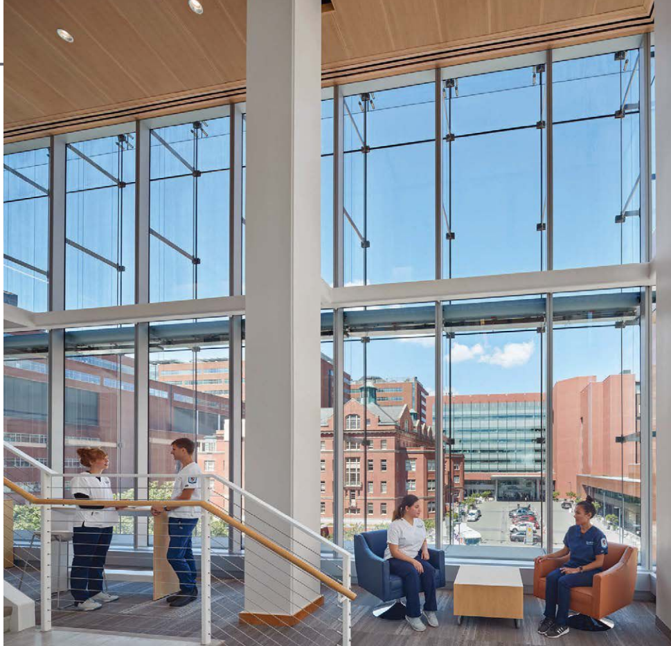
A DOUBLE-SKIN CURTAINWALL SYSTEM AT THE WEST FAÇADE CONTROLS HEAT GAIN, GLARE AND ALLOWS FOR GREATER TRANSPARENCY IN SUPPORT OF THE GOAL OF SHOWCASING ACTIVITY WITHIN THE BUILDING. THIS CURTAINWALL ALLOWS STUDENTS TO GATHER, STUDY AND CONNECT ALONG THE GLASS IN COMFORT.
