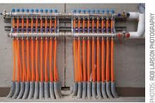
BOTTOM LEFT: THE ESC'S ROOF HOLDS PHOTOVOLTAIC SOLAR PANELS, WHICH CAPTURE THE SUN'S ENERGY TO CONVERT TO ELECTRICITY. TO AVOID ENERGY WASTE, BAT-TERIES INSIDE THE BUILDING STORE POWER THAT CAN BE USED BY THE FACILITY ON OVER-CAST DAYS AND AT NIGHT. BOTTOM RIGHT: COMFORTABLE TEMPERATURES THROUGH THE FACILITY ARE PROVIDED BY RADIANT FLOOR HEATING AND COOLING TIED INTO GEOTHER-
