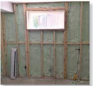
Post flood, drywall is removed and Demilec insulation is intact.
