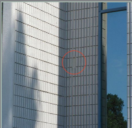
A RECENT PAINTING PROJECT HAD SEALED THE OUTDOOR AIR VENTS TO THE VERTICAL AIR CONDITIONERS, CAUSING TOILET-EXHAUST-INDUCED AIR INFILTRATION TO ENTER THE ROOM AND WALL CAVITY DIRECTLY AND WASH BEHIND THE NEWLY INSTALLED VINYL WALLCOVERING.
