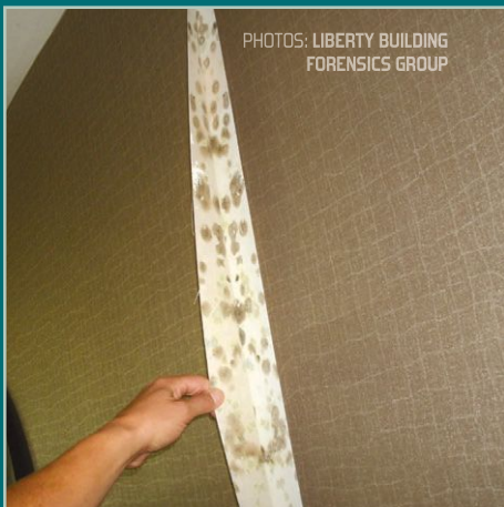
MOLD GROWTH WAS FOUND BEHIND NEWLY INSTALLED VINYL WALLCOVERING AT A RECENTLY PURCHASED HOTEL. THE ROOT CAUSE COULD BE TRACED BACK TO A DECISION MADE JUST BEFORE THE PURCHASE OF THE HOTEL.
