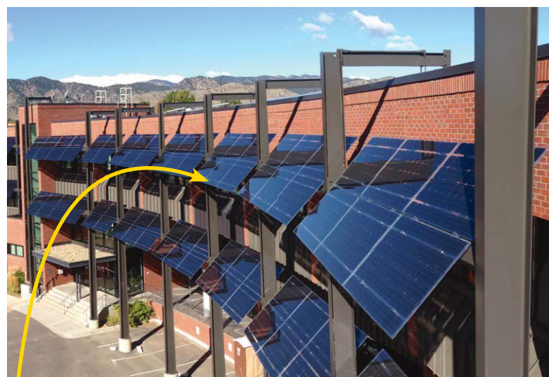
The UCAR Anthes Building, Boulder, Colo., features the LSX Module System from Lumos Solar. The system's through-bolt mounting design and integrated wireway provide design freedom.
