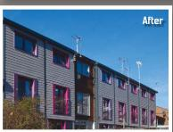
Prefabricated wall panels installed on an existing multifamily building were designed to make the building energy-efficient, warm and desirable to tenants.
