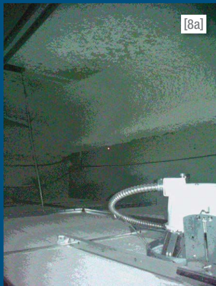
[8a-b] Regular and IR camera images taken above the ceilings reveal a plume of 38 F air (represented by the dark violet color) descending into patient rooms where the exterior walls meet the attic. Note the color scale on the IR image.
