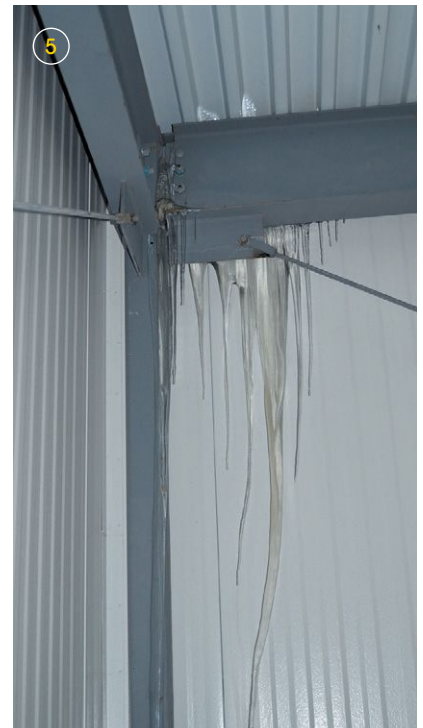
5) Insulation in the roof system is a nuisance, but interior icicle formation, such as this, is a life-safety condition.
