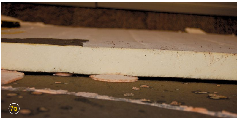
6) Although polyurethane foam is a wonderful adhesive, it must be in contact with the insulation boards to be effective. In this case, the product was not properly mixed and consequently did not rise. This type of workmanship contributed to the roof failure.
