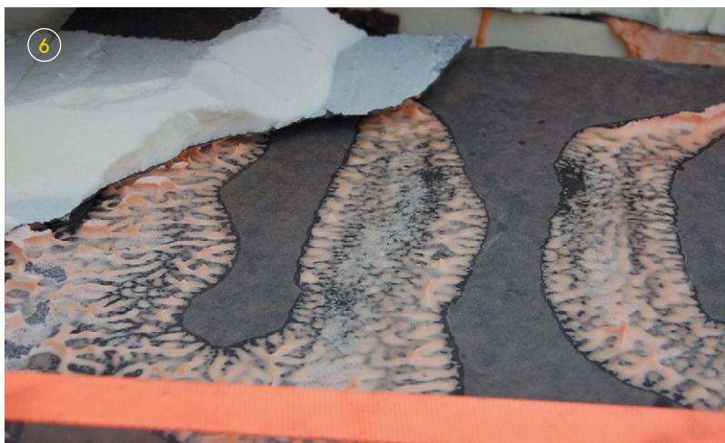
6) Although polyurethane foam is a wonderful adhesive, it must be in contact with the insulation boards to be effective. In this case, the product was not properly mixed and consequently did not rise. This type of workmanship contributed to the roof failure.
