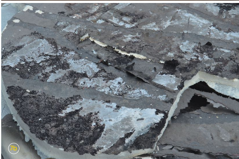
7a) and 7b) Using bead polyurethane foam adhesive can result in the creation of air gaps in the layers of the insulation through which air can pass. Photo 7b shows the result of what happens when warm, moist air meets the dew point. A large medical clinic did not find any solace in the fact that this roof was only one year old and needed to be replaced.
