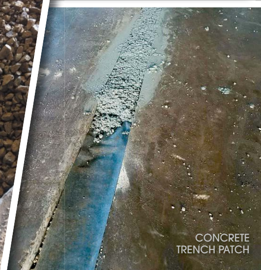
LATERAL TRENCH SAW CUT
