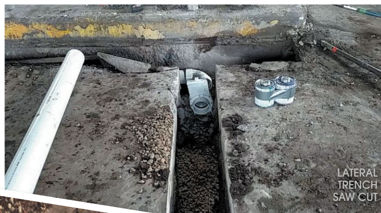
PERFORATED COLLECTION PIPE IN TRENCH
