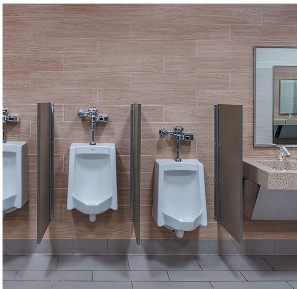
The Corning-Painted Post Area School District in Painted Post, N.Y., now features battery-operated sensor flushometers and Sloan urinals as part of a complete retrofit project.
