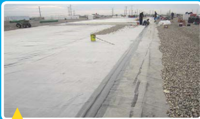
⑤ The new EPDM membrane over new insulation (left) is in the process of being ballasted. The “night tie-in” is easily accomplished with seam tape and self-adhering cover strips.
