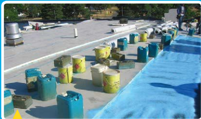
⑦ The blue spray-foam adhesive applied to the existing EPDM is allowed to rise prior to setting the new double-coated, fiberglass-faced, mold-resistant insulation. To ensure positive embedment into the adhesive and bonding, the insulation is weighted in place. The author's spec requires 5- to 35-pound weights per board for a minimum of five minutes.
