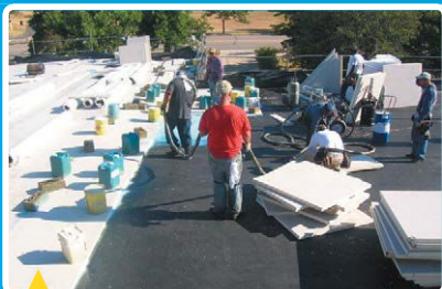
⑥ On this school, the existing EPDM roof membrane is being utilized as a vapor retarder. After cleaning, two layers of insulation are being installed in full-coverage spray foam. The amount of new insulation above the existing membrane was determined by dew-point calculations.
