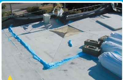
⑧ The roof drains were extended with the new reversible collar pinning the existing EPDM to maintain the integrity as a vapor retarder. A 1/2-inch-per-foot tapered insulation sump is being installed, tapering the top layer of insulation to the new roof-drain extension.
