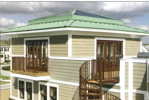
Structural insulated panels, a roof with low-E coating, and electronically tintable glass windows and skylights help to create a durable, energy-efficient building envelope at the Not So Big Showhouse.
