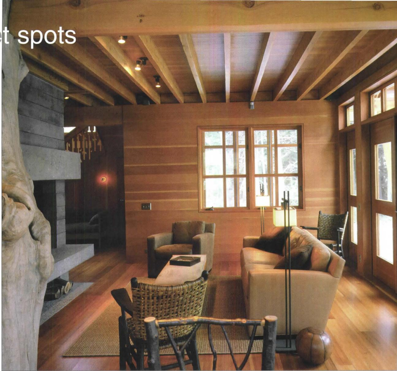
Budget constraints dictated a fireplace made of concrete block. But Bohlin was able to recycle forms from a previous project, and instead they "pre-cast the sections and stacked them like logs."
