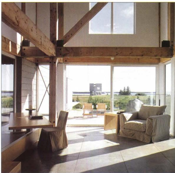
Inside House No. 22, the finger jointing of the “folk tech” frame is exposed (above left). Floating above is the lightweight envelope made of channel-jointed hemlock (above right).
