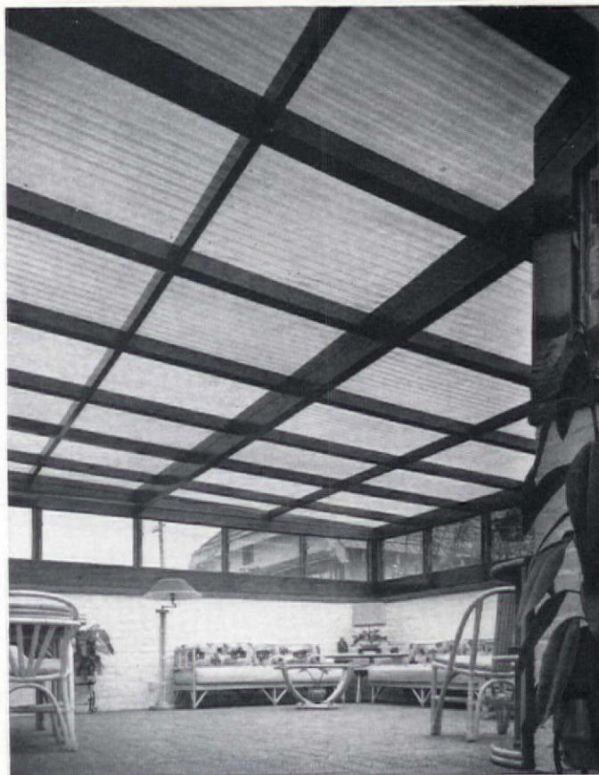
Below: The owners have used plastic panels skillfully to roof this light-and-airy living room. It probably would have been a bit on the dark and gloomy side if they had roofed it with an opaque material
