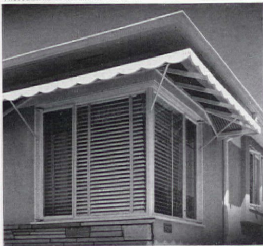
Above: Corrugated panels that top this awning are highly translucent, admit lots of light to the room they shelter. Yet they effectively bar heat
