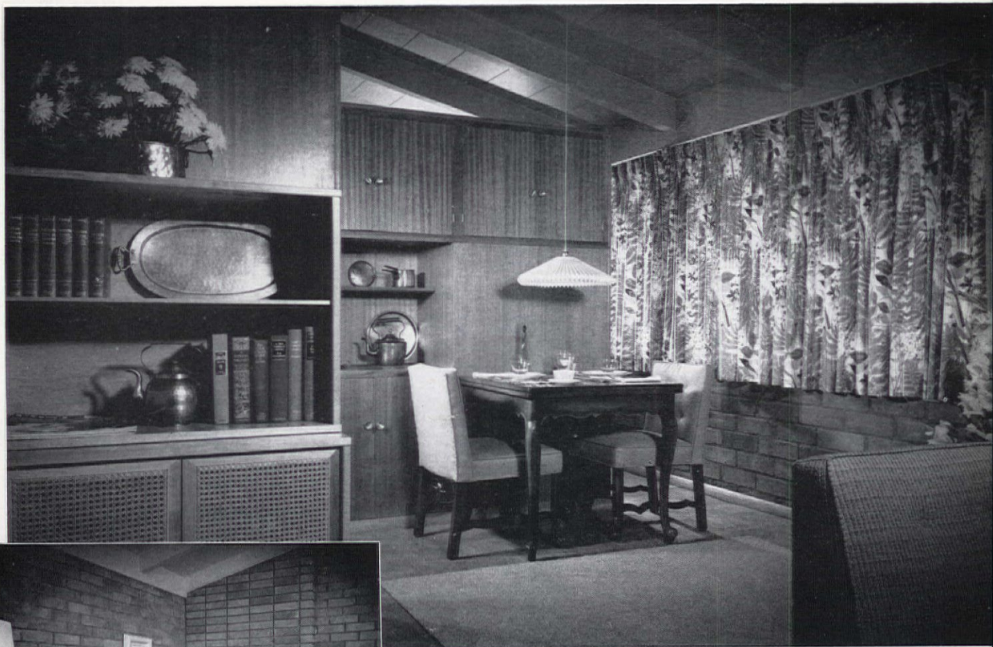
Free-standing storage wall between kitchen and dining area is faced with hardwood.
