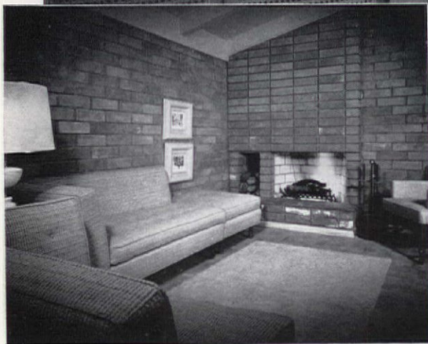
Masonry units of fireplace are laid with aligned joints
