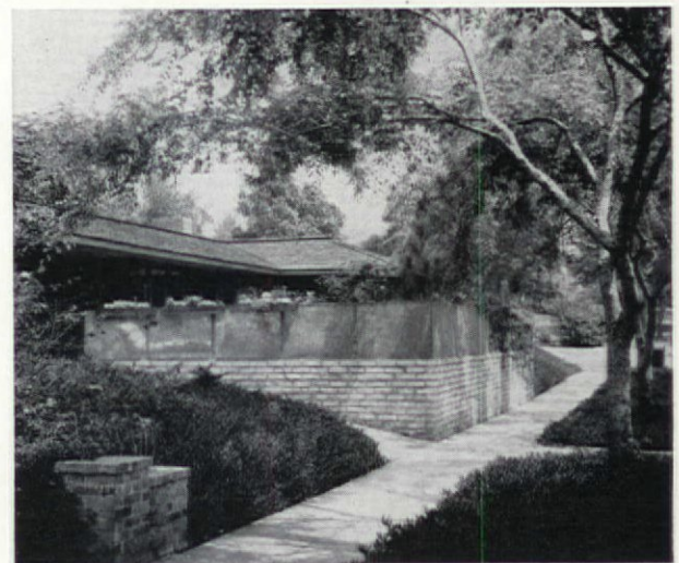
Elaborate use of glass and brick assures privacy within whispering distance of intersecting sidewalks. Less expensive, but equally view-stopping, would be vertical board construction
