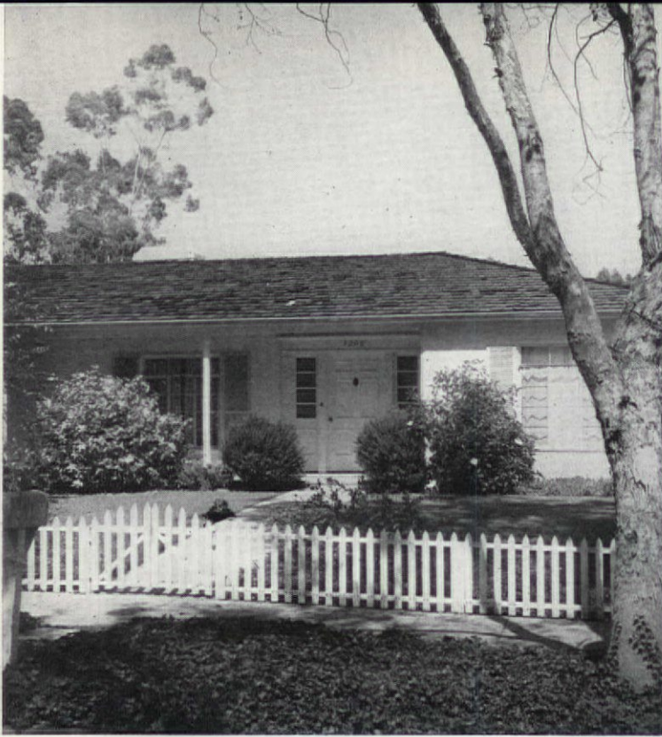
Gateways should never be less than three feet wide. This traditional picket fence is cleft by a simple double gate that swings back and forth at a touch to let family and friends pass through. Tapering line of the pickets is achieved by nailing along rails at graduated heights
