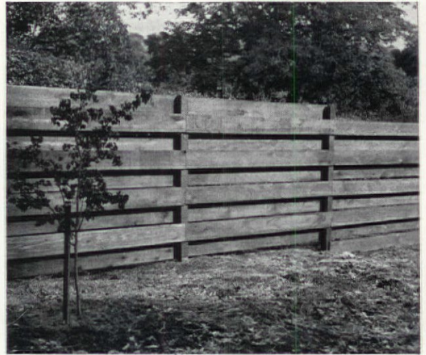
Desire for privacy, undesirable views, protection for livestock are but a few of the reasons for building this horizontal board fence. Note interesting way in which boards are alternated
