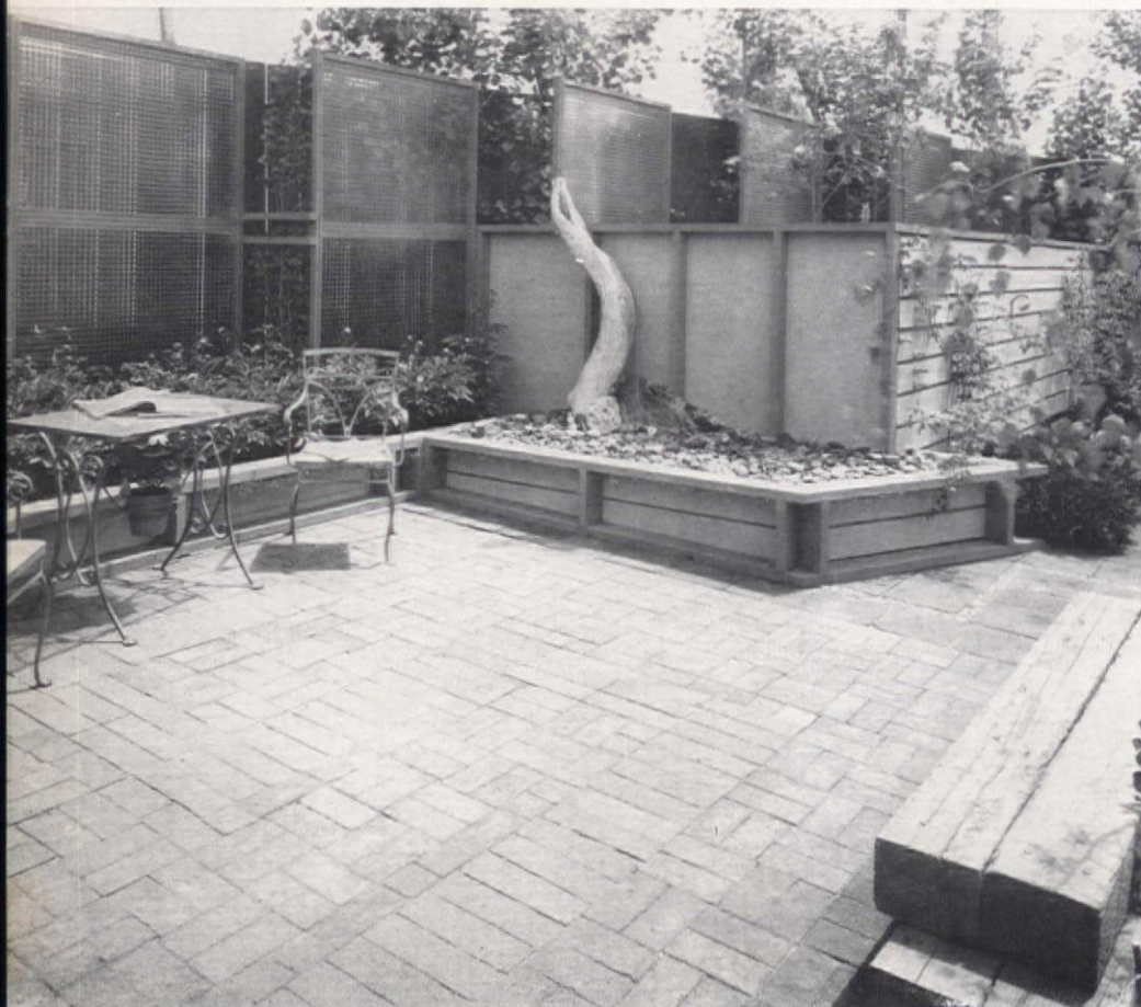
A combination of boards, plywood and patterned glass brings comfort and beauty to this corner
