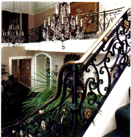
These forged-iron stairs and balcony railing – designed, fabricated and installed by Wiemann Metalcraft for a residence in Wichita, KS, feature a polished-bronze cap rail, rosettes and decorative elements.
