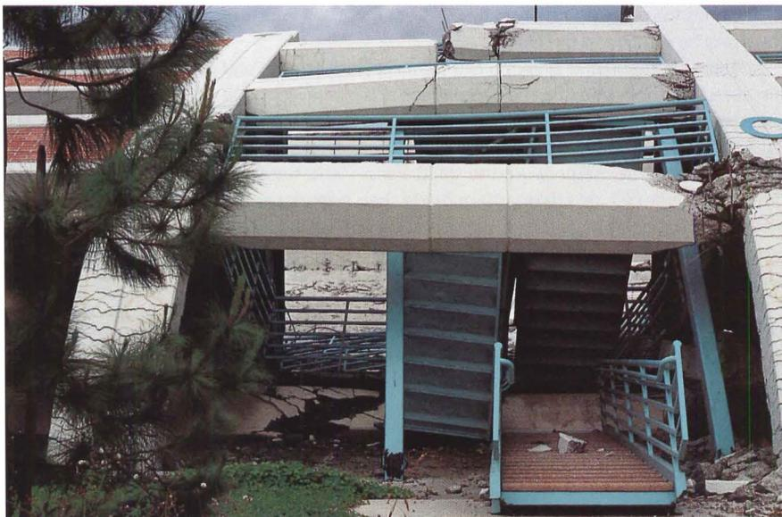
Segments of this precast concrete parking garage at California State University at Northridge fell over, partly because of the garage's long, thin shape and its lack of redundant structure such as interior walls.
