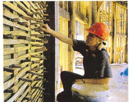
INSTALLATION OF TEMPORARY T-PEGS TO HOLD FIREBOARD IN PLACE DURING THE TUCK-POINTING OF THE PLASTER BEHIND THE OAK LATHS.
