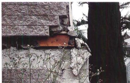
Many buildings with inadequate shear resistance at their base were knocked off their foundations.
