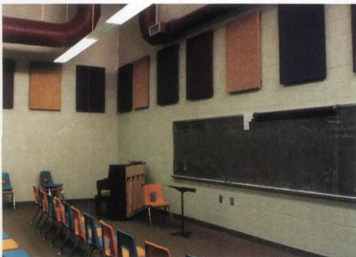
TECTUM PANELS or FABRI-TOUGH fabric wrapped Decor panels to reduce noise in existing or new construction. Colorful, abuse resistant.
