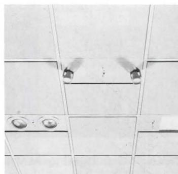
**Exide Electronics:** Ceil-Pak Series, a totally flush emergency lighting system, mounts in t-bar grid ceilings and offers halogen lamps as well as remote units.
