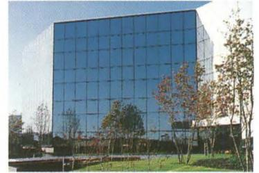
United States Aluminum Corporation is now offering the Series 3200 Curtain Wall system, specially engineered for low and high rise outside glazing applications, to receive 1/4" or 1" glazing.
