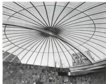
**Rolladome** is a motor-driven operable dome skylight of galvanized steel with bronze acrylic glazing. Opening the skylight vents heat buildup in summer, and single glazing allows maximum solar gain in winter. Rollamatic Roofs, Inc.
