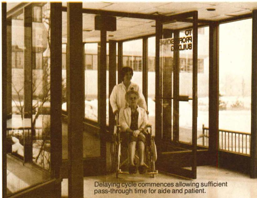
Delaying cycle commences allowing sufficient pass-through time for aide and patient.
