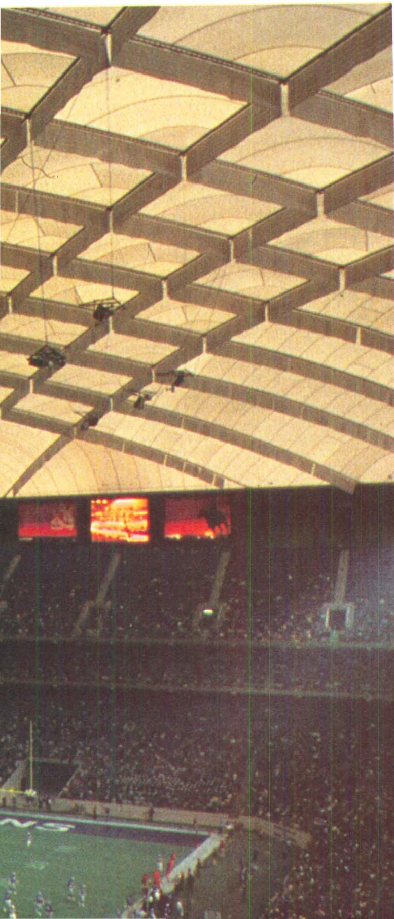
An air-supported dome of lightweight Fiberglas® coated with DuPont TEFLON® fluorocarbon resin completely roofs Pontiac Silverdome, home of the Detroit Lions, Detroit Pistons and Detroit Express. The 10-acre area is the largest permanent structure roofed with architectural fabric to date—and the stadium cost far less to build than comparable stadiums using other dome approaches.
