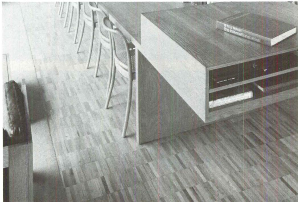
Among recent innovations in resilient flooring is the development of acrylic-impregnated (and also vinyl-bonded) natural wood and cork flooring, which has the appearance of its natural components and the ease of maintenance and durability of its synthetic ones. PermaGrain acrylic/wood flooring is used in Kent Memorial Library, Suffield, Ct, by Warren Platner (right).
