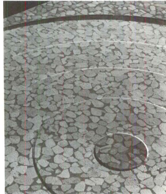
Two solutions to pattern wearability problem include choosing an inlaid flooring (such as Armstrong's Corlon, above right), in which pattern extends into entire thickness of material, or specification of a solid-color, raised-pattern flooring (such as Norament by Nora Flooring, above left).
