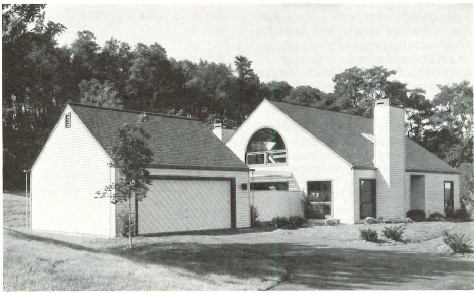
Painted aluminum siding was used on exterior rather than oxidizing aluminum panels architect wanted. Living room (below) is separated from family room (below right) by kitchen.
