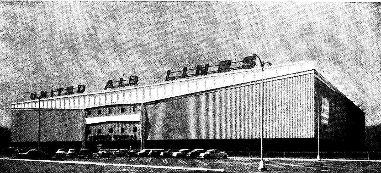
United Air Lines Service Center at San Francisco, Cal. Mahon Metal Curtain Walls were employed to lend trimness and to retain the clean lines of this unique structure which was designed to accommodate four mammoth DC-8 Jet Air Liners. Mahon Curtain Wall Plates, of the same material and pattern, were also employed as exterior facing on the large hangar doors.
