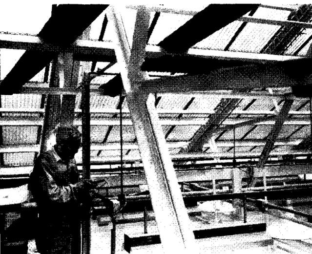
*Figure 1—Presently being reconstructed, Wing E of the Metropolitan Art Museum will ultimately have an electrical and lighting installation comparable to Wing J. Workman (above) connects two conductors above the T-grid in Wing E.*
