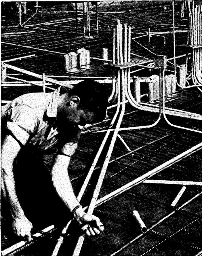
**GOOD INSTALLATION PRACTICES** call for tying Republic ELECTRUNITE E.M.T. to steel rebars. With steel conduit there is no danger of galvanic action.
