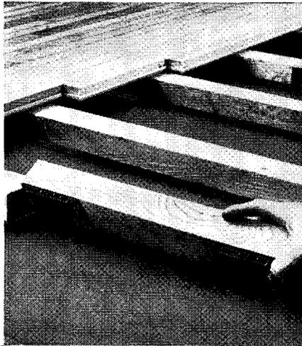
The secret is in PermaCushion's patented design which features an extra-thick maple floor system floating on resilient pads. The floor is not attached to slab, walls or other structural members — remaining permanently smooth because it can expand and contract without buckling or cupping. The air-channeled pads cushion the entire floor, preventing shin splints and improving play. PermaCushion stands the test of time — its unmatched resiliency and smoothness last for generations.
