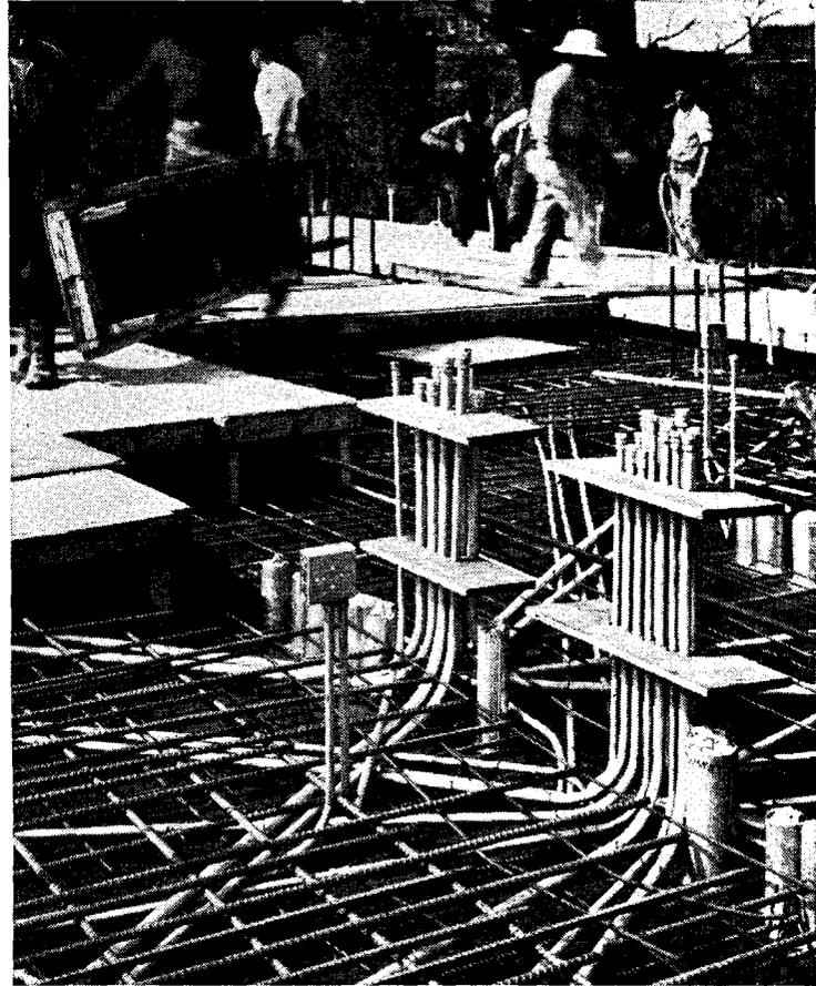
**ELECTRUNITE "INCH-MARKS"®** and **"GUIDE-LINES"®** help make compact stub groupings. The strength of steel provides protection against damage.
