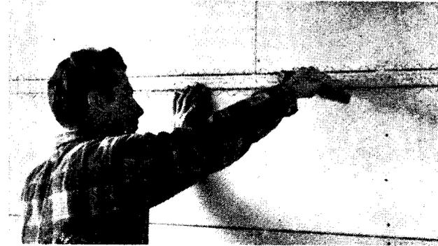
KEYSTRIP can be used as a reinforcement for plaster in a space too narrow for strips of gypsum lath. A full bond of Keystrip to the plaster is assured. Keystrip also adds strength to points of stress above doors and windows.
