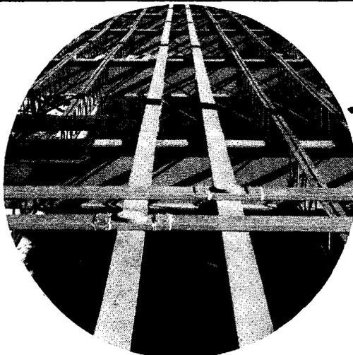
This construction view shows the clean arrangement of header ducts installed on Ceco E/C Joists. These header ducts were installed quickly and economically by an electrical crew which had never before installed a system of underfloor electrification.
