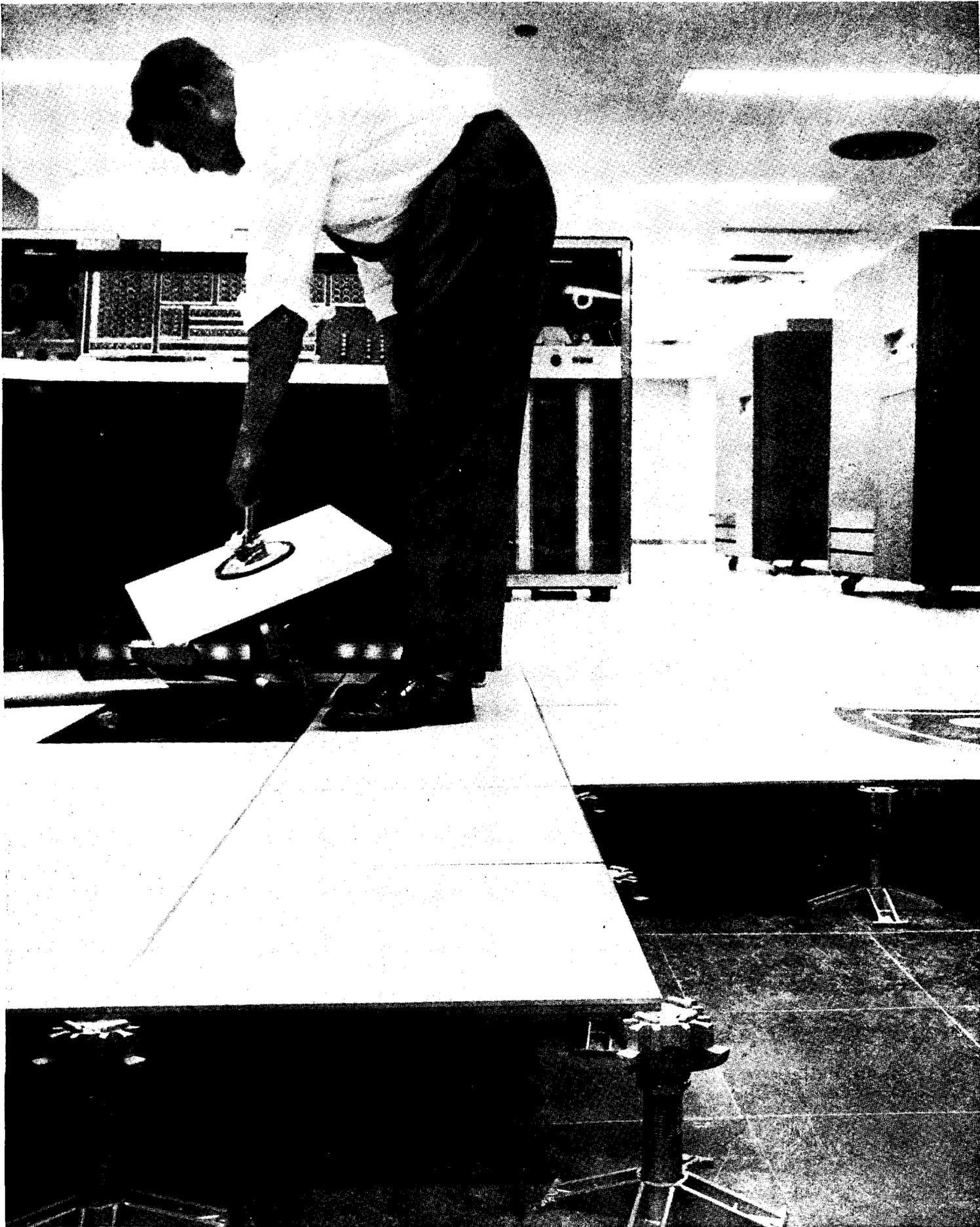
Complex network of cables seen during installation of a large-scale IBM computing system will be completely concealed by an elevated floor of Alcoa Aluminum. This installation is at the office of United Medical Services, Inc. (New York's Blue Shield).
