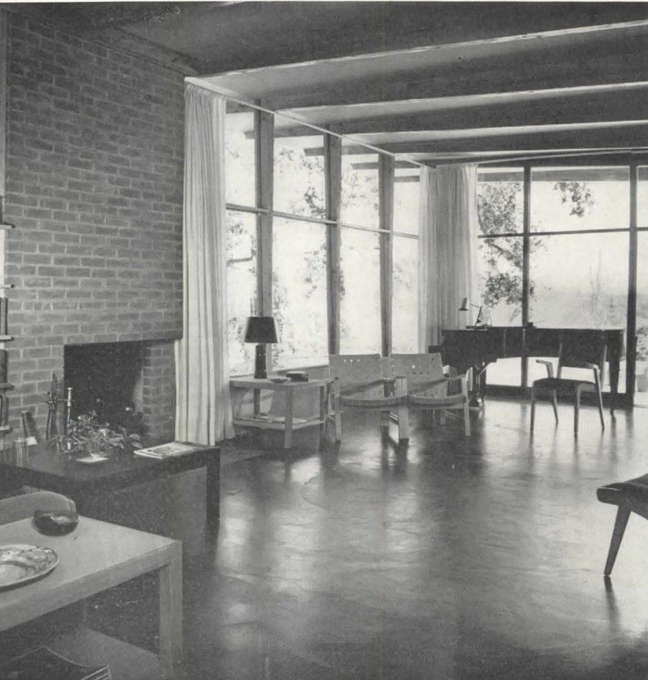
*Interior wall surfaces are of striated plywood on stud frame; the cement floor is integrally colored. The house has a radiant-heating system in the floor slab. The black pattern on the floor plan indicates the vertical elements of the structural system.*
