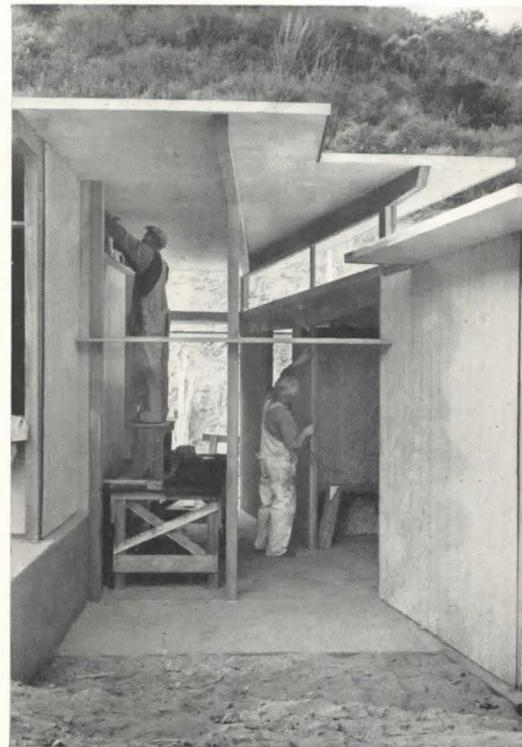
*The independent structural frame (left) permits any sort of enclosure within reason. On a sloping site, the system can simply be stepped down hill (above), the roof break allowing introduction of a clerestory window. Roof edging is stainless steel.*
