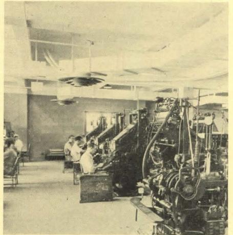
Figure 5—overhead outlets supply air to composing room containing linotype machines.
