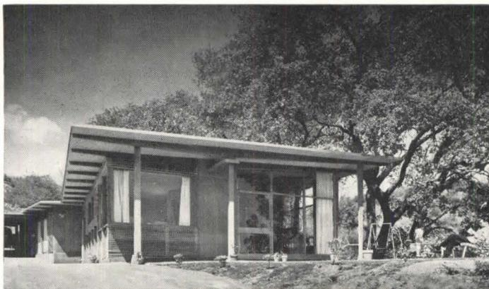
*The pattern of the rafter frames, fixed glass, and louvered ventilation areas is clearly shown in the porch-end view of the completed house. The bedroom detail shows a combination of fixed glass, tilt-in wood sash, and in-opening plywood panels beneath that serve the ventilating louvers.*
