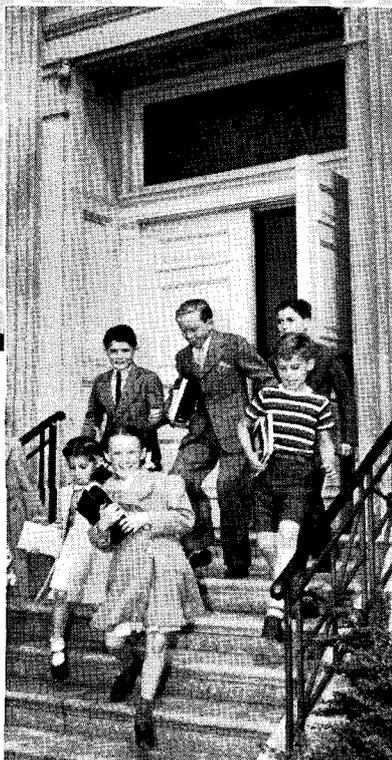
**4** RIXSON UNI-CHECK operating classroom door leading out of doors. Classroom floor is elevated two inches to prevent driving rain from entering. Uni-check is imbedded into lower level. This treatment is suitable only in warm non-freezing climates.
