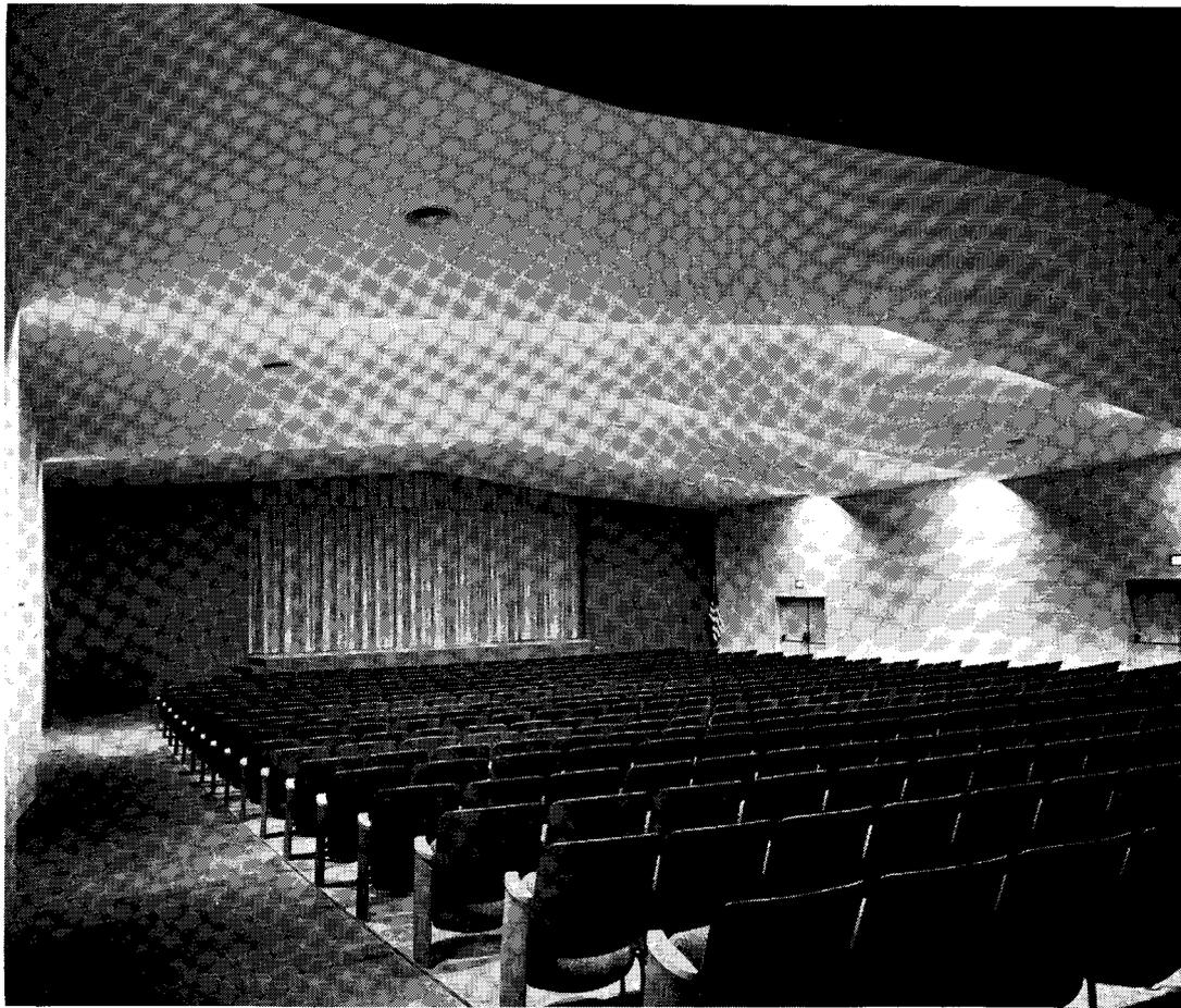
*Both the walls and the ceiling of the auditorium have broken sections, which, with the semi-absorptive surfaces and glass-fiber-blanketed rear wall, provide acoustic correction. Side walls and ceiling are light gray; the front wall is dark green; and the rear wall is rose. Figuring covered area at one half, the cost of the building came to \$9.50 per sq ft.*
