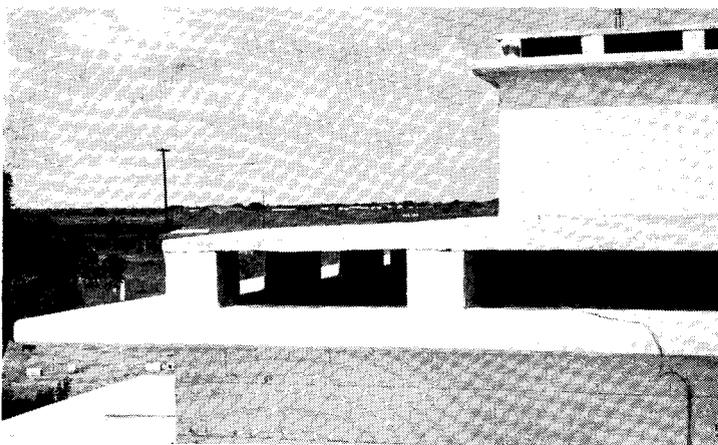
Figure 7—concrete double roof at Kano, Nigeria. Upper slab provides protection against solar radiation.
