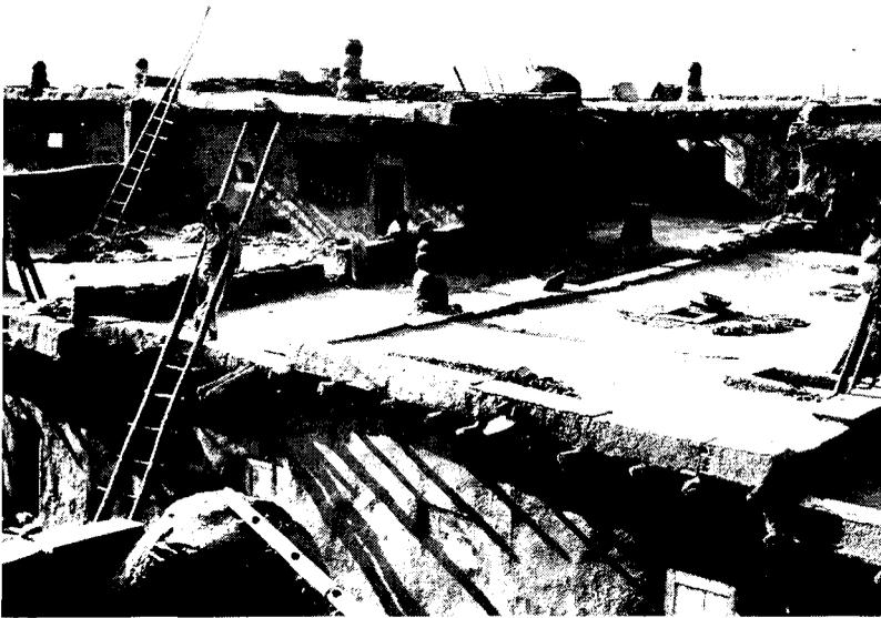
Figure 3—thick earth walls and roofs of Pueblo Indian houses in hot-dry New Mexico produced small openings and deep reveals; in addition, a longer time was required for sun heat to penetrate to the interior surfaces.
