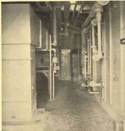
Figure 2—fan room in mechanical building contains newsroom air-conditioning system (right) and composing room system (left).
