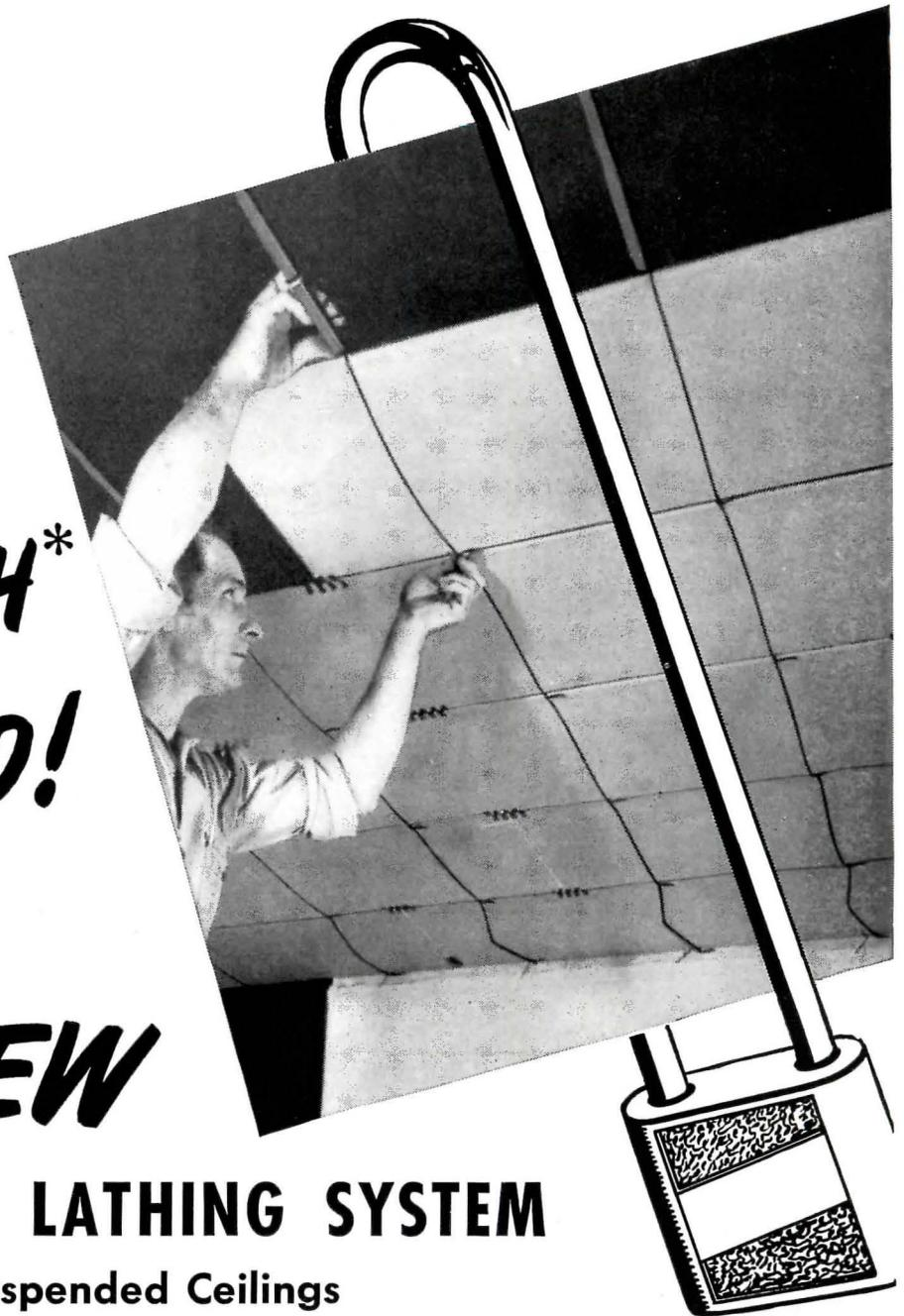
USG's new BRACE-TITE Lathing System gives you all the advantages of ROCKLATH plaster base—plus the desirable features of suspended ceiling construction. It is easily adjusted to the contractor's working methods because no special tools are used, and no time-consuming training is required for either lathers or plasterers.
