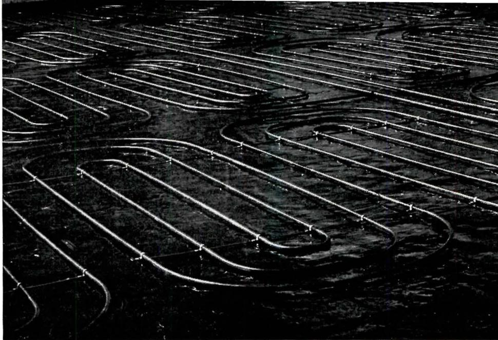
EVEN-RAY COILS BEING INSTALLED: left, single coil, showing spreaders; right, auditorium floor.
