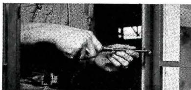
If the casements are being erected in wood construction, the screws should be applied so as not to distort the casement frames. For instance, screws are never drawn tighter in one hole than in another.
