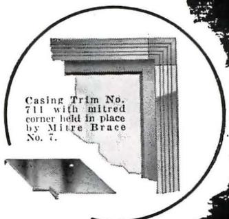
Casing Trim No. 711 with mitred corner held in place by Mitre Brace No. 7.
